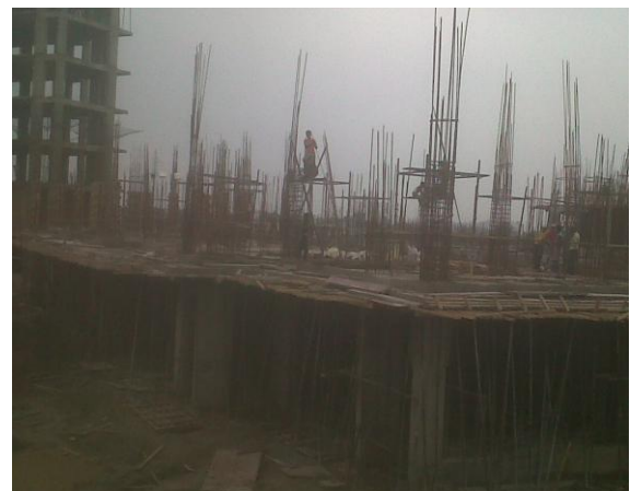
Tower F (Above Basement Slab Column Casting in Progress)
