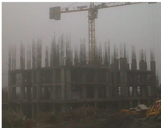
Tower E (2 nd Floor Slab Shuttering in Progress)
